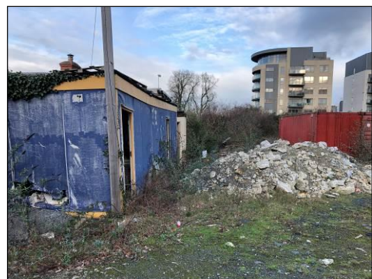
Plate 6.4 - Example of portacabin structure.
